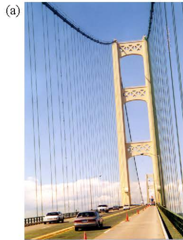
Cables of Mackinaw bridge
